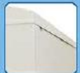
movable roof for maintenance
